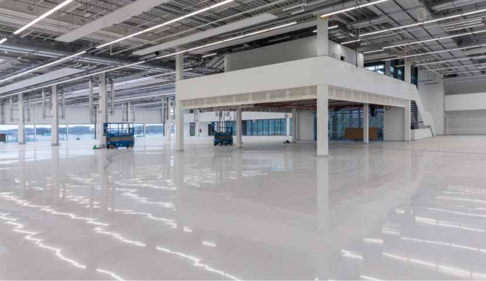
The future production space offers ample room for business growth.
