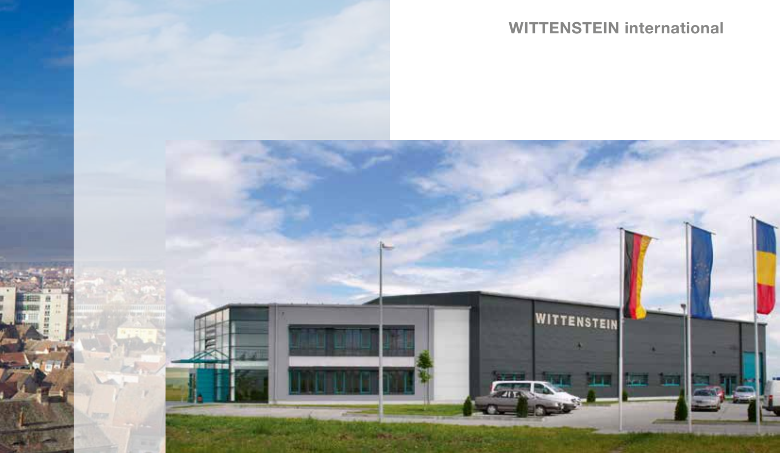
The WITTENSTEIN manufacturing plant in Șura Mică opened five years ago.
